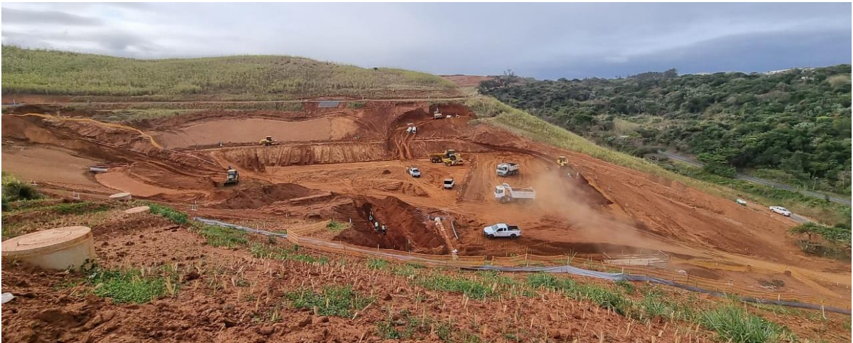
Photo above: Node 5 attenuation pond under construction (30/08/2021)
