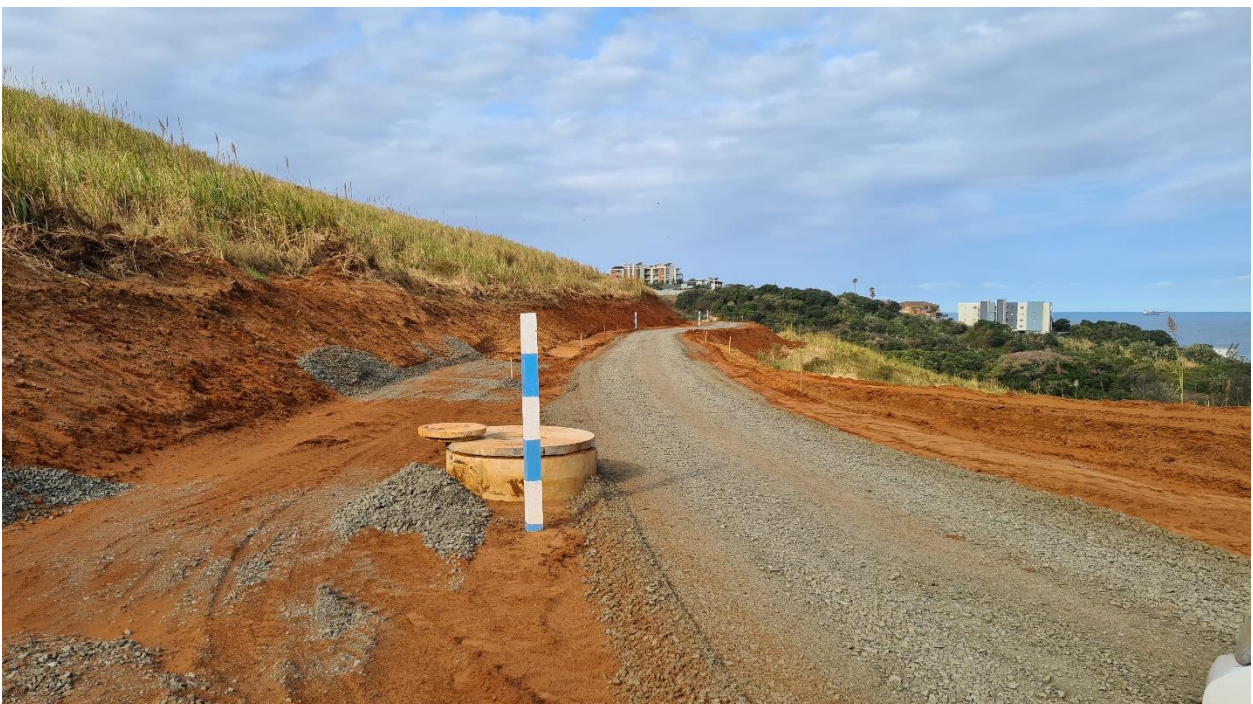
Photo above: service road on gravity main through Node 5 (30/08/2021)
