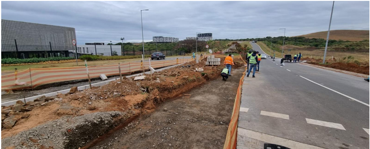
Photo above: Circle 6 modification underway (05/08/2022)
