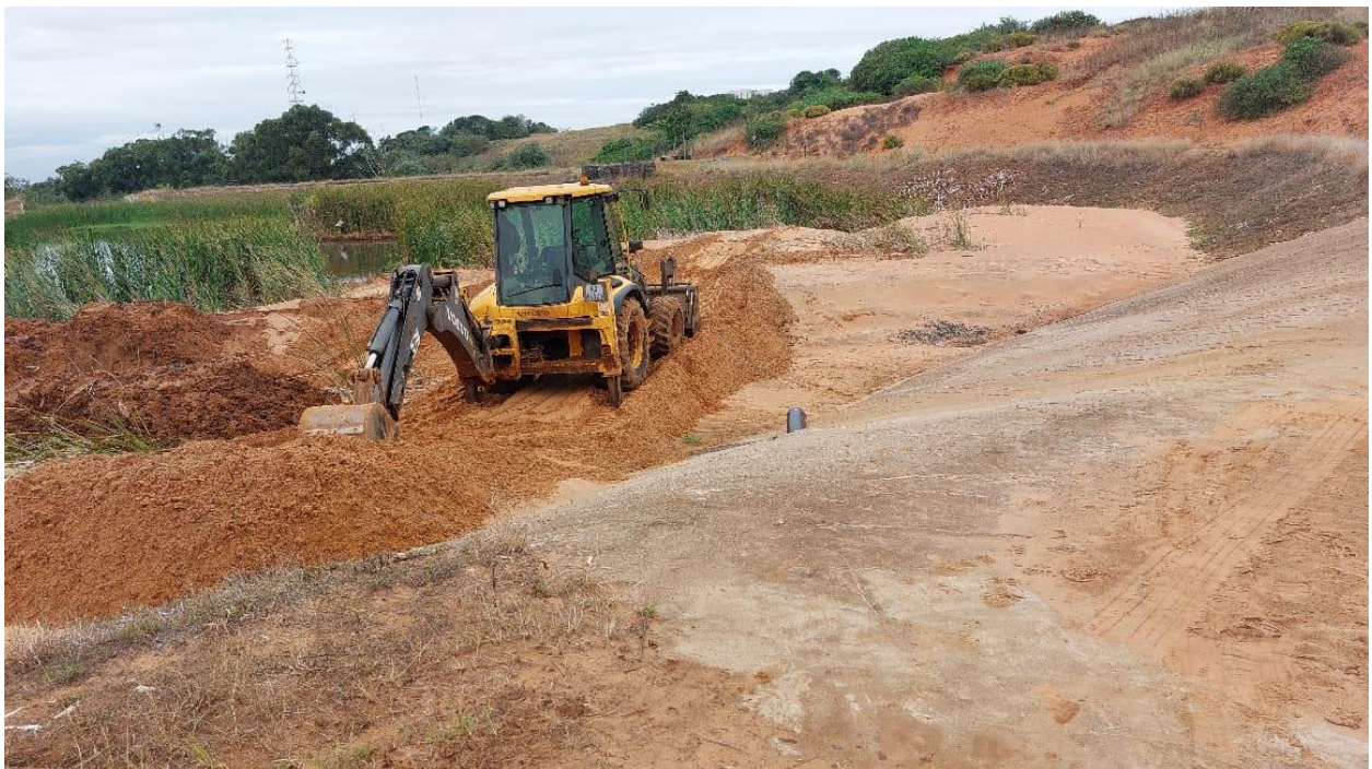
Photo above: Infrastructure teams attending to de-siltation of Pond 1 (07/2022)
