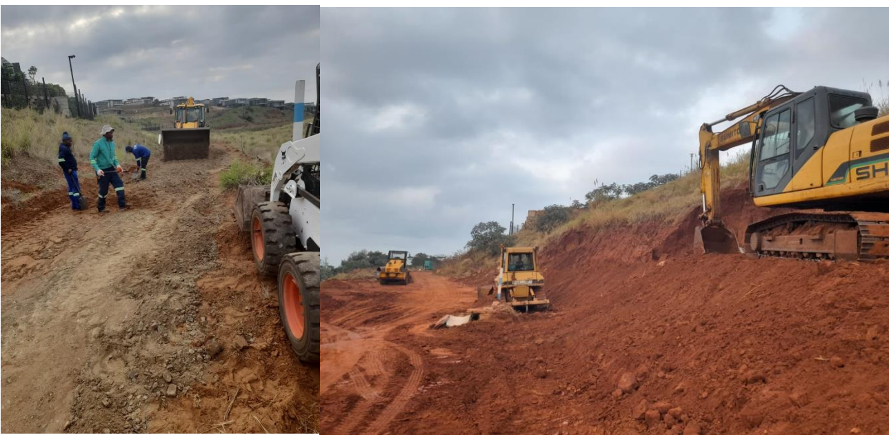
Photo above: Remedial work to access road from Heleza Blvd as well as ongoing remedial work to Services servitude in node 5.
