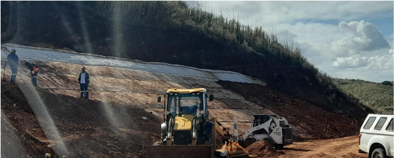
Photo above: Remedial work to scour above node 5 services servitude ongoing and making progress.
