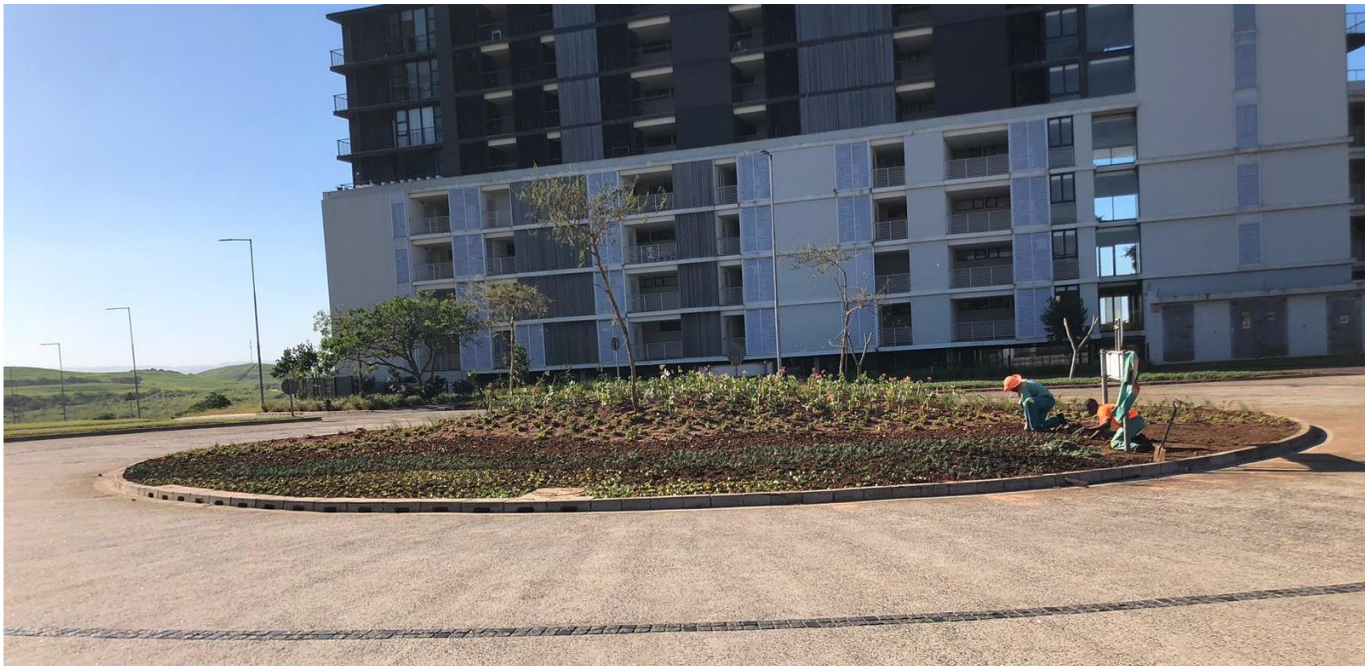
Photo above: Circle 4 During the implementation of the Landscaping Special projects being completed.
