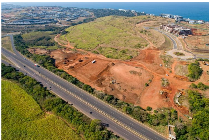
Photo above: Work underway on the commencement of Heleza Blvd extension and the new retail centre platforms early September.
