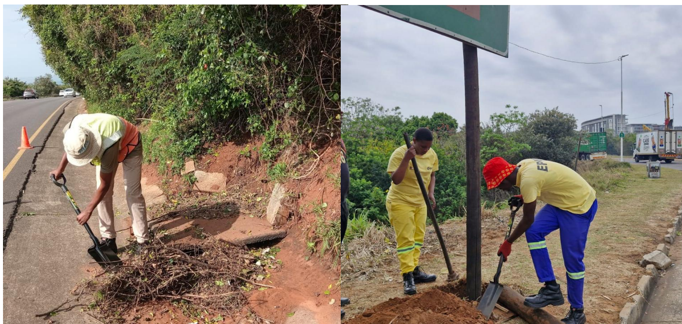
Photos above: Maintenance teams attending to supplementary cleaning of M4 Storm water infrastructure and DOT teams repairing signage following requests for maintenance.
