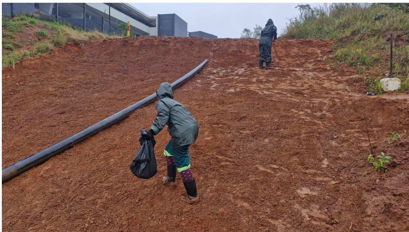
Photo above: teams seeding recently repaired and reinstated storm water civils in node 5.
