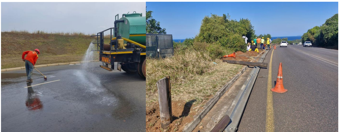
Photos above: Clean up operations following a concrete spill on Heleza Blvd following a penalty instituted against an errant contractor and DOT teams attending to Guard Rail replacement following requests
